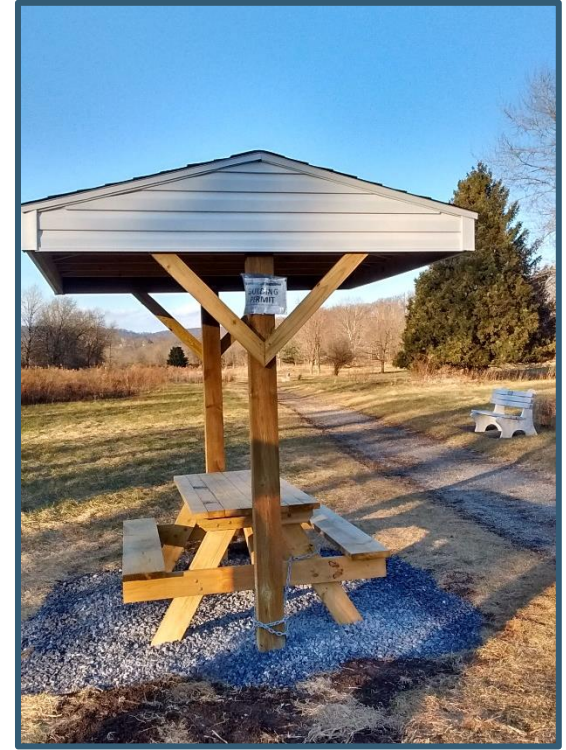
Covered Picnic Pavilion at the Vincent DiFilippo Nature Preserve Completed in 2016 by Matthew Lawrence
